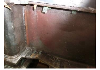
(b) without weld access hole
