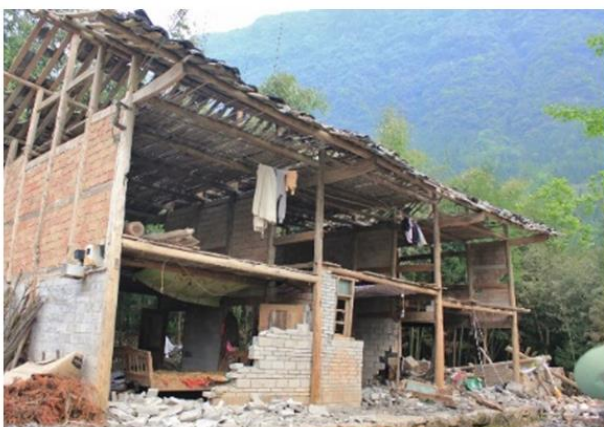
(a) Chuandou timber frame after Lushan earthquake. (Qu et al., 2015)
